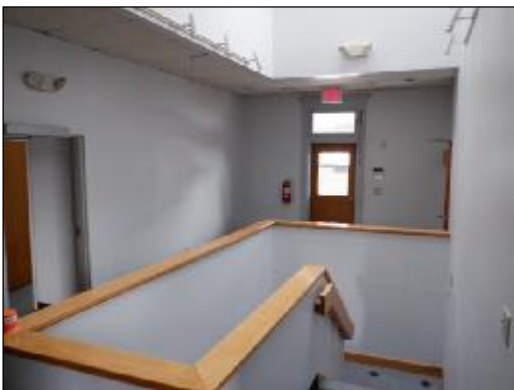
Interior, As-Is – 2 nd floor, stairwell and landing, looking SE
