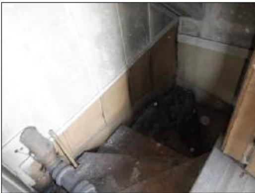
Interior, As-Is - attic, stairs
