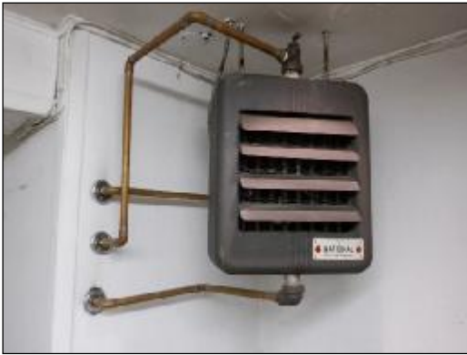
Interior, As-Is – basement, overhead space heater
