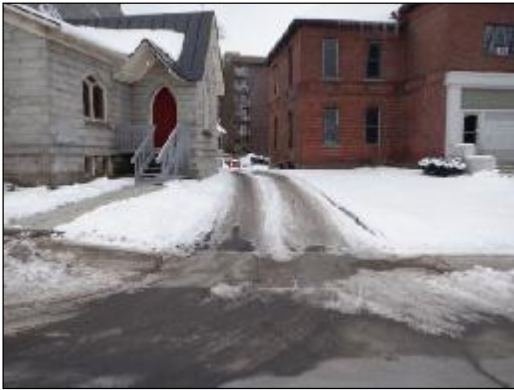
Site – access drive, looking S from Church Street
