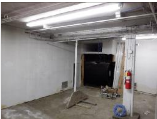
Interior, As-Is - basement, looking E
