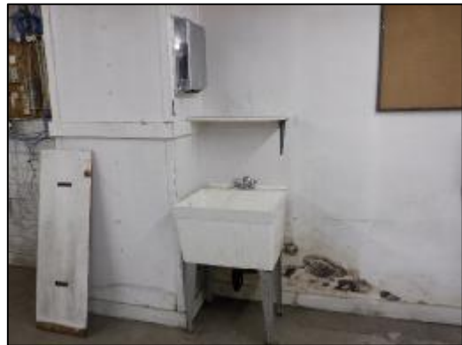
Interior, As-Is – basement, slop sink
