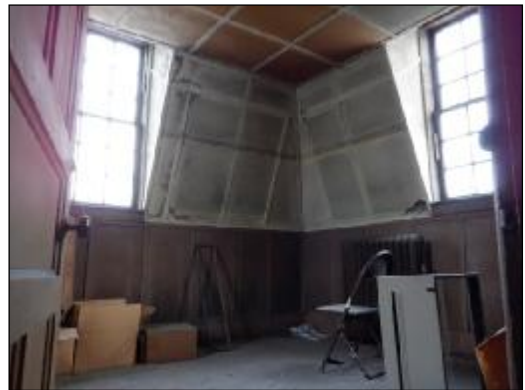
Interior, As-Is - attic, looking NE
