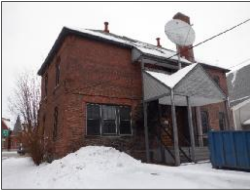
Exterior, As-Is – SW corner
